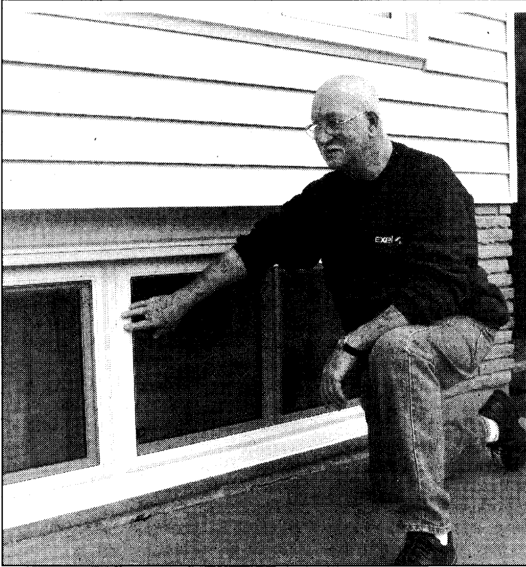
John McRobbie shows one of the brand new basement windows that was recently installed at his home on Aaron Drive.
